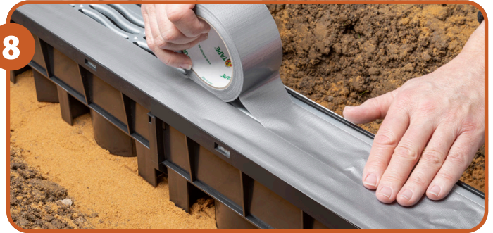
8 Protect grate with tape before concrete is poured.
