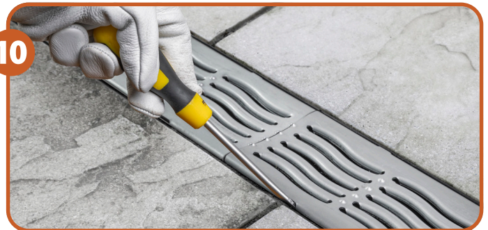
10 Insert a screwdriver into the slots provided, twist and lift to remove the grate.
