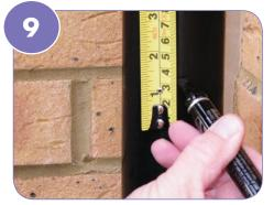
Mark 30mm/38mm/70mm\* above the level line on the downpipe.
