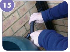
Attach the flexible hose to the diverter.
