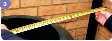
Make sure that the water butt is positioned no more than 500mm from the downpipe.
