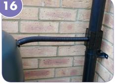
Attach the flexible hose to the water butt connector.
