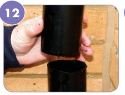
Remove the cut section.
