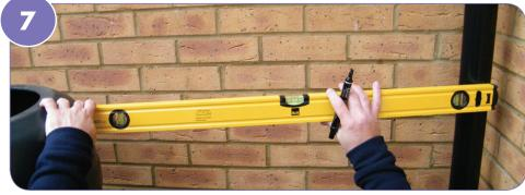
Use a level, positioned at the bottom of the your drilled hole.
