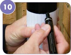
Handy tip: use a piece of paper around the pipe to get a straight line.
