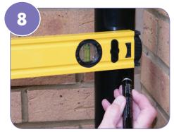
Mark a level line from the bottom of the hole on the downpipe.
