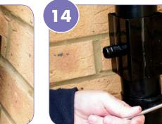
Attach a pipe clip to support the diverter.
