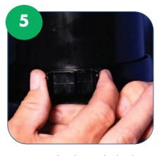
Squeeze the clips at the back together to secure the Strap on Boss to the soil pipe.
