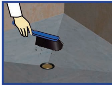
11. Dust the cement floor.
