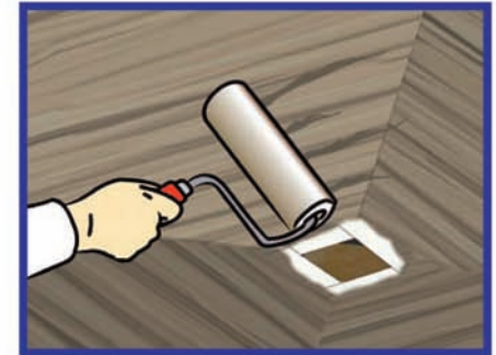
15. Put a new layer of watertight resin on the strips and over the concrete then leave to dry.
