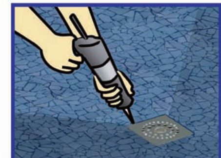
21. Create a seal between the grid and tiles using a silicone mastic.
