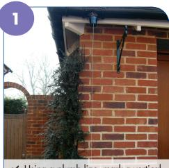
✓ Using a plumb line, mark a vertical line on the wall from the outlet to the drain.
