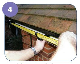
✓ Mark the position of the fascia brackets, spacing them no more than 1000mm apart (400mm in areas of heavy snowfall) and no more than 150mm from any angle or stopend.
