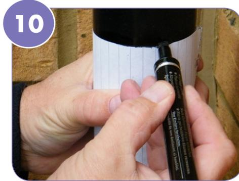
10 Handy tip: use a piece of paper around the pipe to get a straight line.
