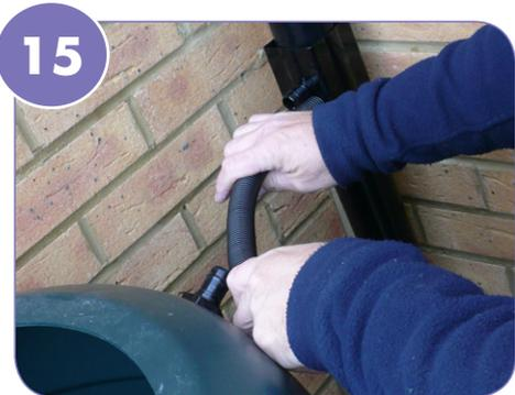
15 Attach the flexible hose to the diverter.
