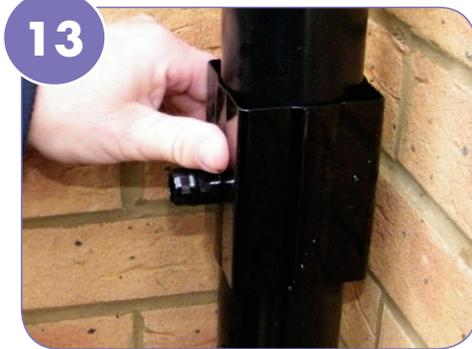
13 Manoeuvre the diverter onto the downpipe.
