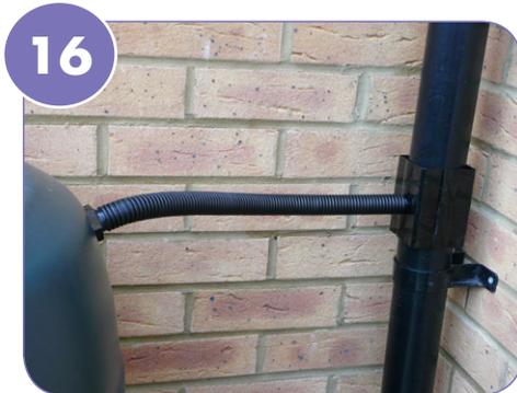
16 Attach the flexible hose to the water butt connector.
