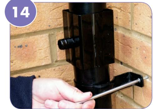
14 Attach a pipe clip to support the diverter.
