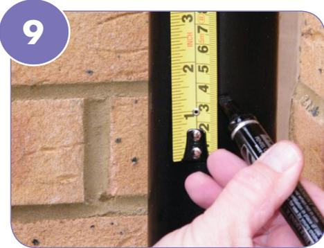
9 Mark 30mm/38mm/70mm\* above the level line on the downpipe.
